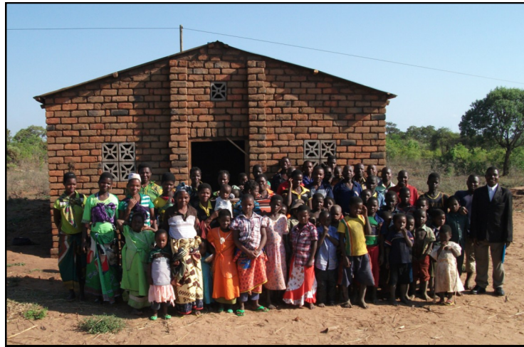
Nondwe Prayer House in Mozambique, recently provided with iron sheets by zm
